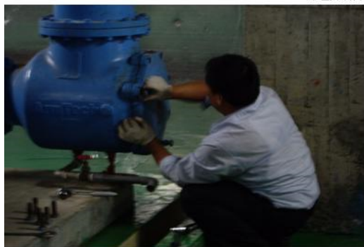
(1)拆卸過濾網蓋板
